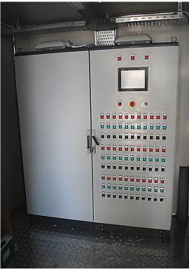
Electric board, IP 54 is suitable to contain the power, control, monitoring and alarm devices for the plant. The controls shall be identified by metal plates fixed by screws. All instruments shall be safety anchored and located so as to keep proper geometry, both horizontally and vertically.
